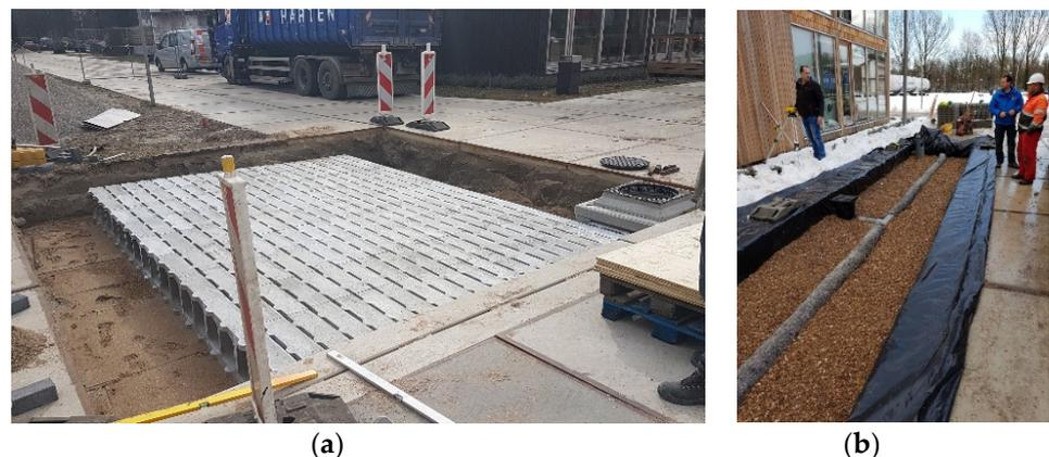
Figure 2. Examples of permeable systems that were full-scale tested at the Urban Living Lab Green Village TU, Delft, the Netherlands: (a) Bufferblock system, (b) Urban Rainshell.
