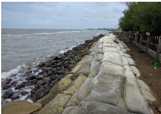
Figure 9, protection of the coast of kota Pekalongan against erosion by sandbags
