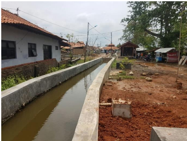
Figure 30, pipes are made in the side to allow water to flow in the canal during floods
