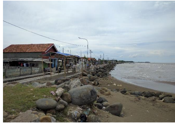
Figure 8, coastal protection without the use of sandbags
