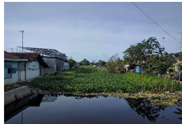
Figure 10, water hyacinths are blocking the flow of the water in canal Bremit
