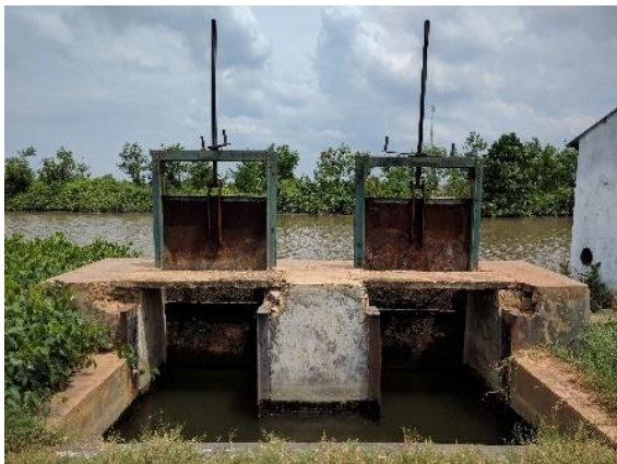
Figure 17, intakes are open during the day when drainage using gravity is possible. Fishponds are drained to river Meduri
