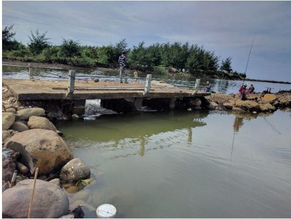
Figure 21, gate where water is able to flow into the fishponds during high tide. Gate is marked in figure 22
