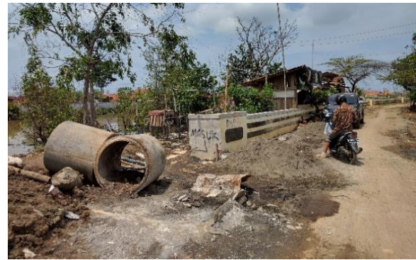
Figure 14, the flood defence wall in kabupaten Pekalongan next to river Meduri ends at the border with kota Pekalongan
