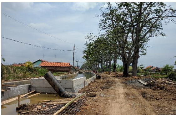
Figure 13, the drainage canal to river Meduri in kota Pekalongan ends at the border with kabupaten Pekalongan
