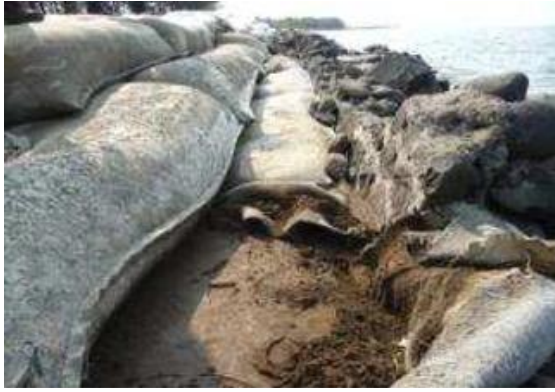
Figure 7, damaged sandbags for the coast of kota Pekalongan (Wilms, 2016)
