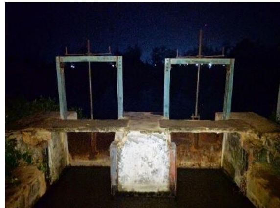
Figure 18, intakes are closed at night when the river Meduri is too high to drain water from the fishponds
