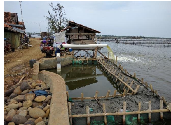
Figure 24, water is drained on the fishponds in the North of sub system 4 by using a pump
