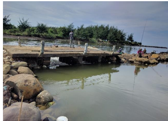
Figure 6, bridge where water flows into the fishponds during high tide
